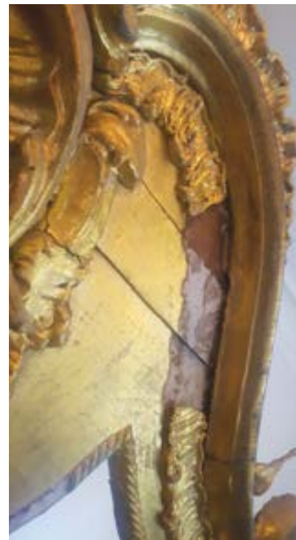
Above: A close look at a damaged mirror frame
